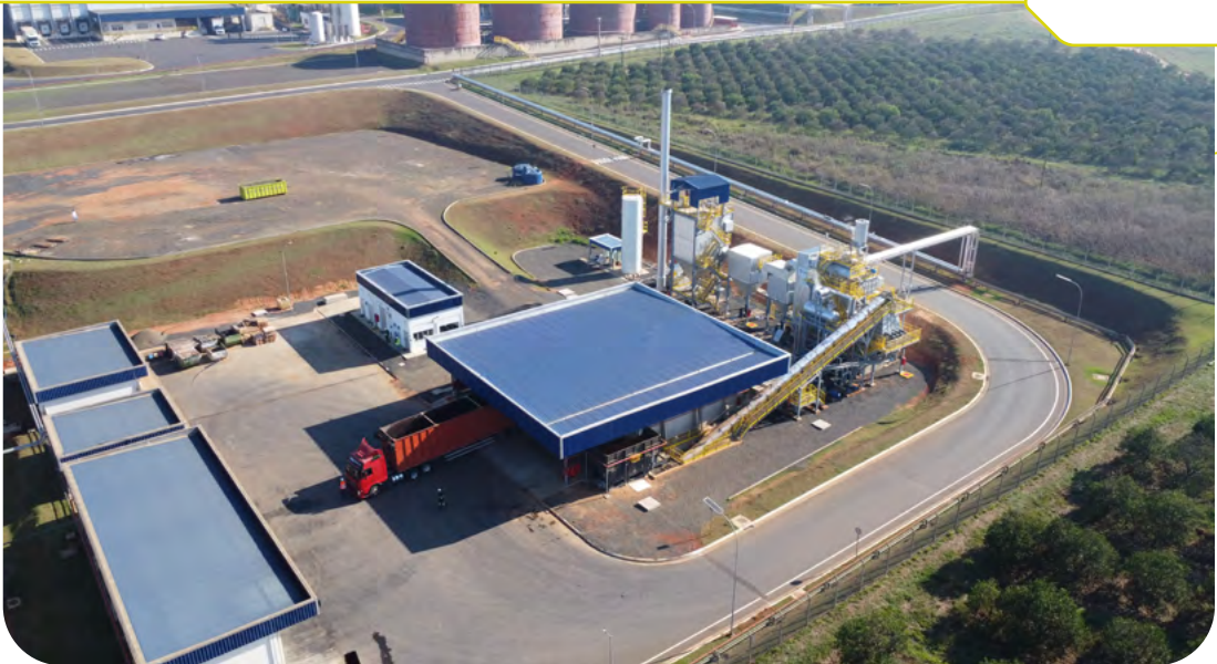
Biomass-fired thermal power plant.
